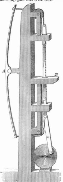
The tension with which the saw is strained depends on the stiffness of the spring, which, of course, can be regulated at pleasure. As the saw moves up and down the spring vibrates back and forth on its pivot, always keeping up the same strain. The stuff to be cut is fed against the saw, at B, in the usual manner. Motion is given to the saw by pitman C.
