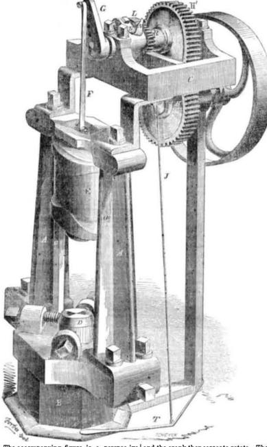
The accompanying figure is a perspective and the crank then ceases to rotate. The drop, iew of the patent Drop Press (with its recent | E, is now at the head of the fall, ready to deimprovements,) for which a patent was grant- scend, but a spring catch, not shown on the ed to Milo Peck, of New Haven, Ct., on the 28th Nov., 1851, and which was illustrated on page 140, Vol. 7, Scientific American.
