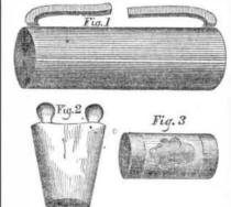
The annexed figures represent two inventions of Capt. J. Norton, of Cork, Ireland, for the purposes specified in the above caption. Fig. 1 is a perspective view of a railroad fog signal, and fig. 3 is its igniter. Fig. 2 is the device for blasting the stumps of large trees.
