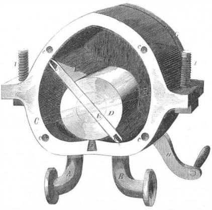
The accompanying figure is a side view- which a patent has been applied for by Josein perspective, with a plate of the casing re- phus Chandler, of Attica, Ohio. These are for the purpose of receiving the moved—of a Rotary Pump and Engine, fo
